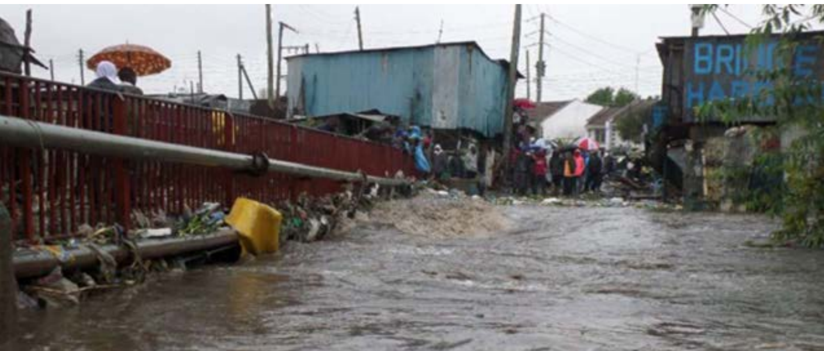
Figure 16 Hazina/Kaiyaba bridge flood Source: Daily Nation
